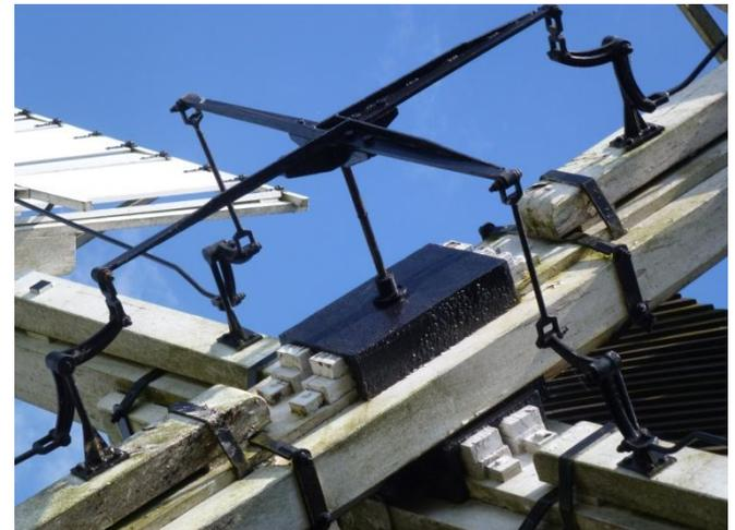
Patent Sails. The vanes are lifted and set from within the windmill, and the amount showing is dependent on the wind speed.
